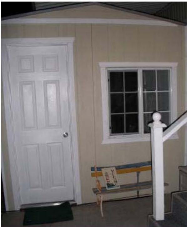
The finished cottage!
