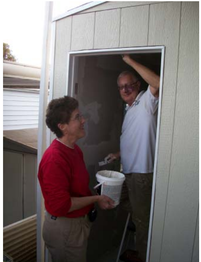
Debby and Gary doing the messy job--taping and mudding the drywall!
