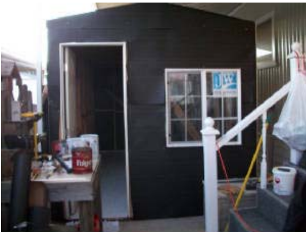
All wrapped in paper ready for siding and roof and trim.
